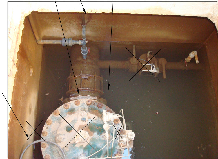
EXISTING PUMP CONTROL VALVE EXISTING PUMP CONTROL VALVE CUT AND CAP REMOVE EXISTING PIPING AND VALVES
